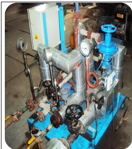
Figure 7.6 Steam Heating System
